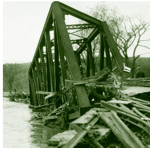
Montpelier 1927, CVRR Bridge
