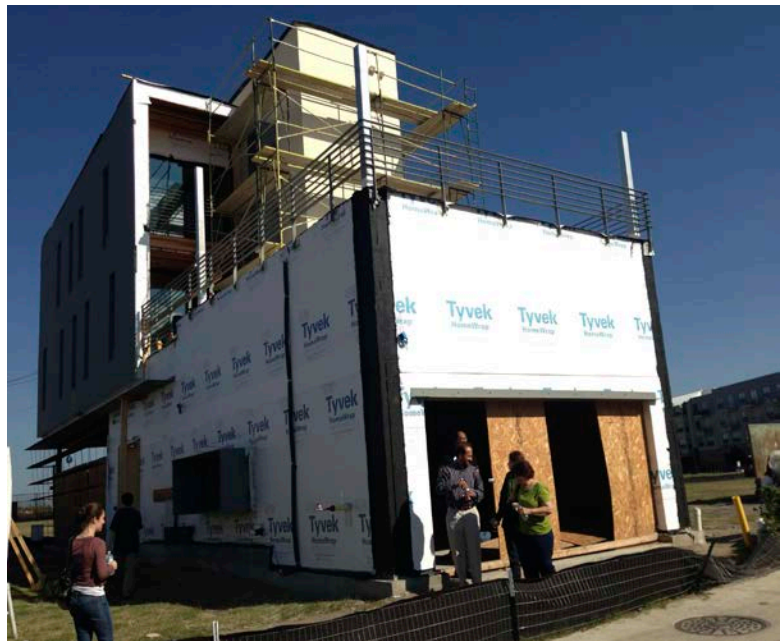
Pike Powers Lab under construction in the Pecan Street Project's Mueller neighborhood in Austin, Texas.
