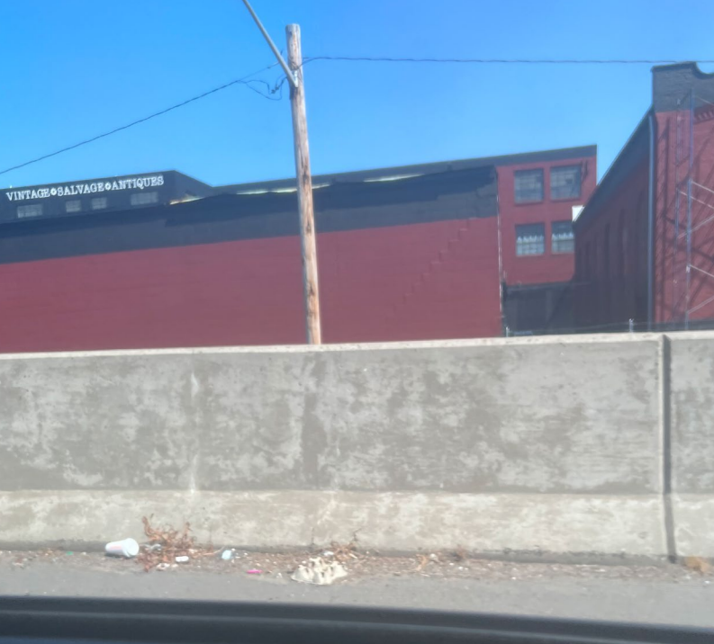
Bridgeport Roadway near housing
